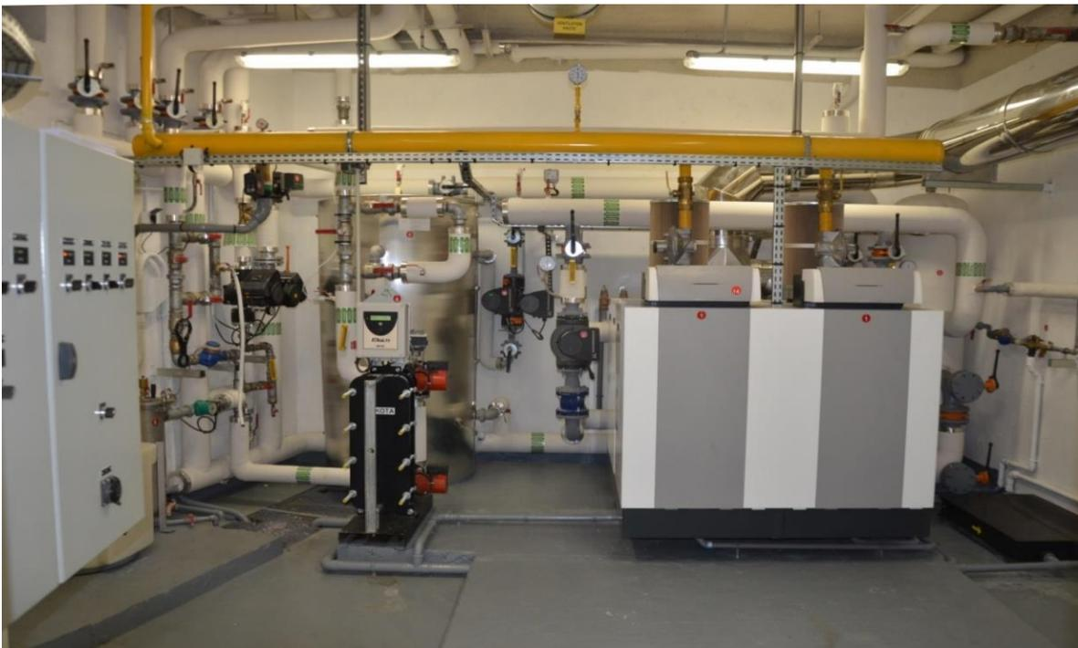
The two holes to connect the condenser of the aquathermal heat pump are provided on the return circuit of the radiators (see right of the photo)
