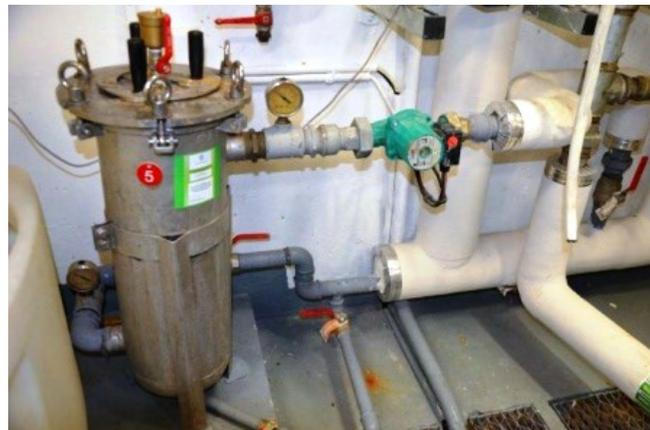
*Filtration fine circuit chauffage*
